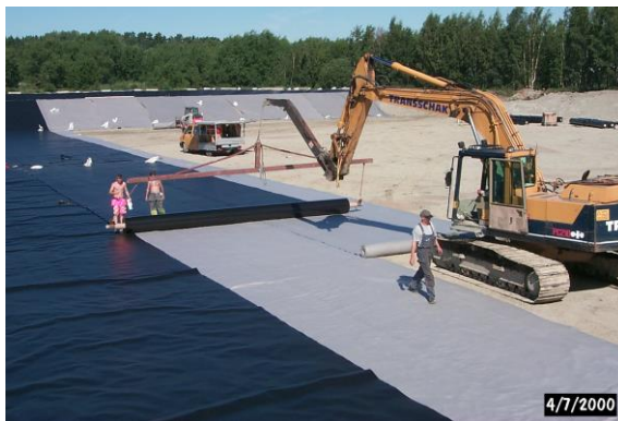
Lined ponds for winter storage
